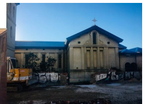
The wall is almost down...
